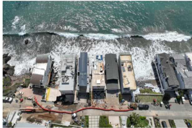
A sinkhole is seen on the street and driveway of a seaside home affected by recent heavy surf on Sea Level Drive in Malibu on Sept. 12, 2026, in Los Angeles. The city of Malibu declared a local emergency and issued evacuation orders for 31 homes after a massive and expanding sinkhole opened up in the driveway of Cage's oceanfront residence. IRYU/VCG VIA GETTY IMAGES
